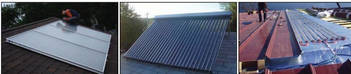
**Figure 2. Solar Collector Technologies Analyzed in the Assessment; the technologies pictured are (left-to right) flat plate, evacuated tube, and building-integrated**
