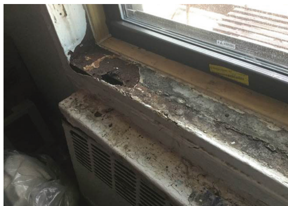
Photo 8: Rotting and corroding window lintels, peeling and chipping paint, as well as rodent feces.
