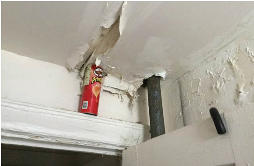
Photo 9: Due to extensive water damage to the ceilings and walls of this Bronx cluster site, the bathroom of this unit was collapsing in. A Pringles can was used to keep the ceiling from collapsing on the tenants.
