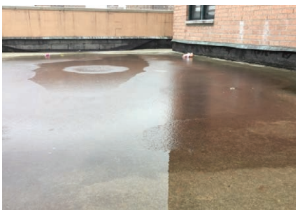
Photo 7: Facility-wide water damage that was likely the result of the failing roof. Flashing in disrepair and water pooling up on the roof indicated improper drainage.
