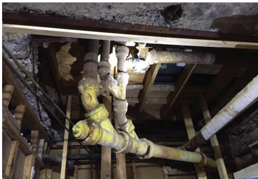
Photo 10: The exposed bottom of a bathtub in a Bronx cluster site where broken 2x4s were used to support it. Had the tub fallen it would have landed on the building's main gas line.
