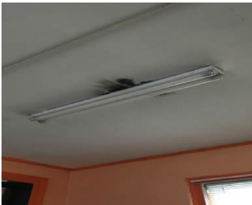
Photo 4: Burn marks near a lighting fixture indicated electrical failures and a serious fire hazard.
